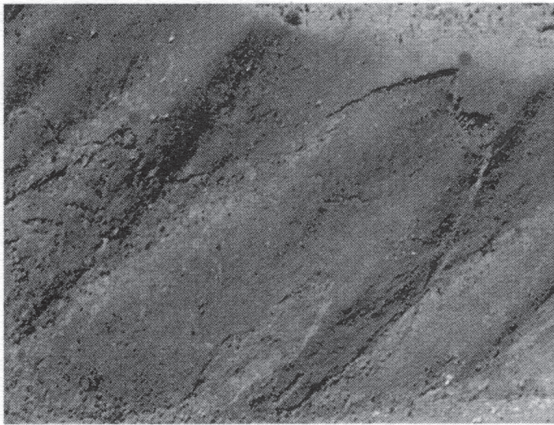
(a) Ma On Shan landslide site
